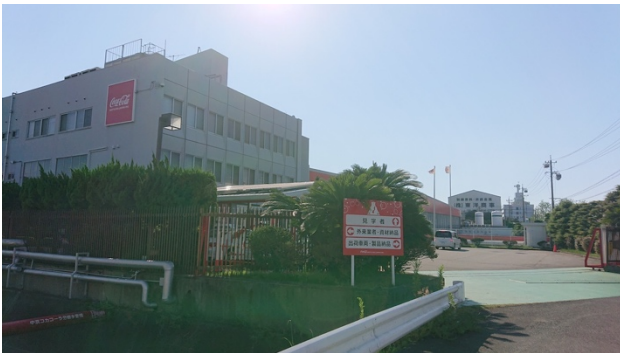
Fig. 1 Coca-Cola Tokai Plant
